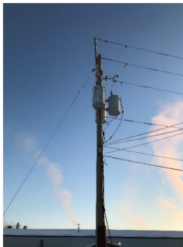
Figure 3.1. Existing Pole Mounted Transformer
