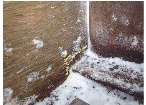
SU1 Ballast wall - NE. Note: Mechanical spall behind G6 bottom flange.
