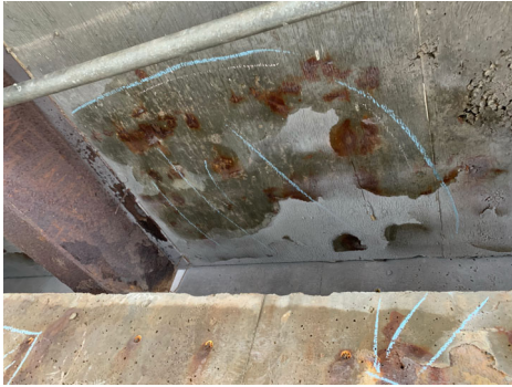
Deck Soffit - Interior - SU1. Note: Typical delamination.
