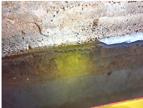
Culvert North Footing. Note: Disintegration and erosion of footing with exposed rebar.
