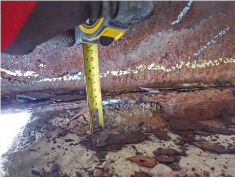
G2 @ SU1. Note: Severe section loss on the bottom flange.
