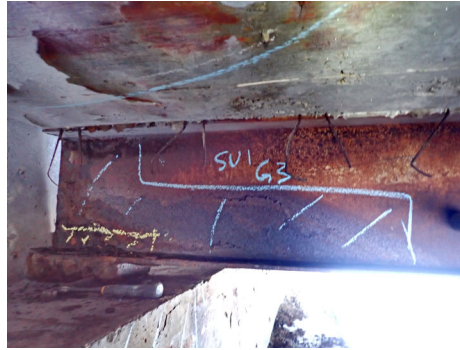
G3 @ SU1. Note: Typical corrosion.
