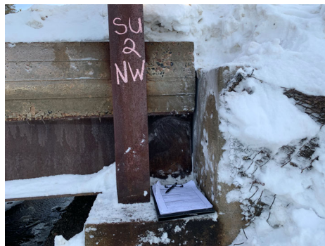
Foundation - NW. Note: Gap between deck top and ballast wall at SU2.
