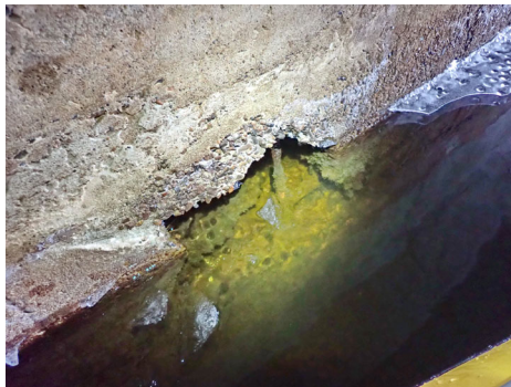
Culvert South Footing at midspan. Note: Disintegration (~450mm deep) of footing with exposed rebar.
