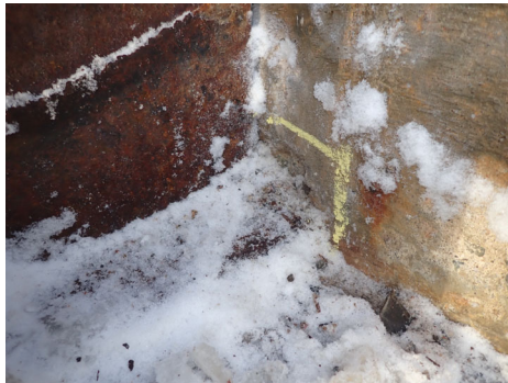
SU1 Ballast wall - SE. Note: Mechanical spall behind G1 bottom flange.
