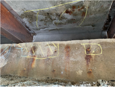
SU1 Abutment wall. Note: Typical delamination and rust staining.
