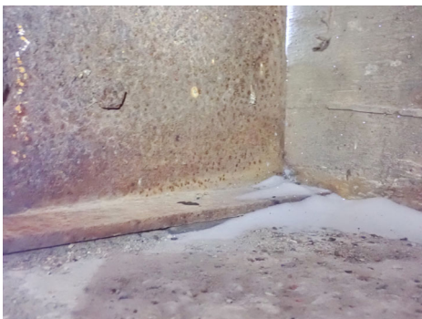
Typical exterior bearing - SU2.
