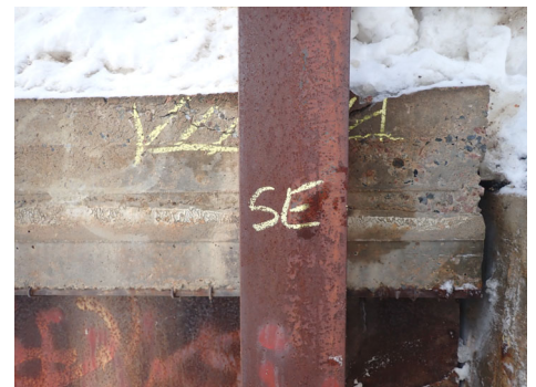
Deck Soffit - Exterior - SE side. Note: Spall behind post.
