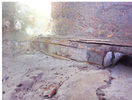
Typical interior bearing - SU2.
