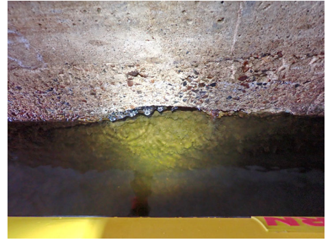
Culvert North Footing. Note: Disintegration and erosion of concrete footing with exposed rebar.
