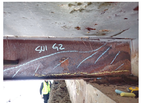
G2 @ SU1. Note: Typical corrosion.
