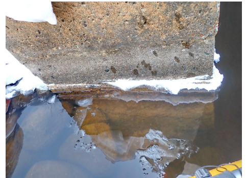
Outlet - SE corner. Note: Disintegration and erosion of concrete footing.
