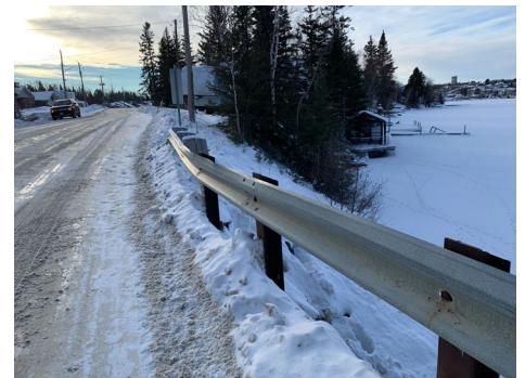
Railing - North. Note: Permanent deformation.
