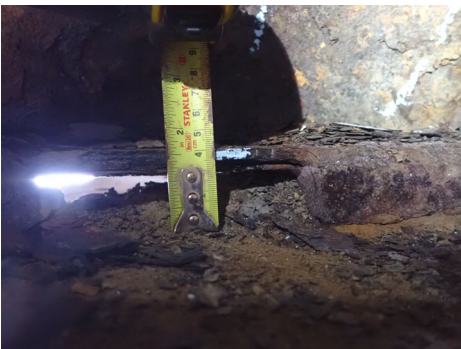
G5 @ SU1. Note: Severe section loss on the bottom flange.
