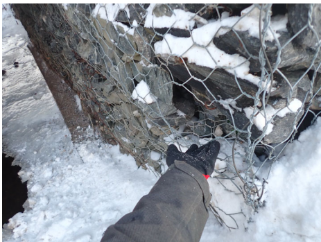
Slope Protection - SU2. Note: Typical hole in wires.
