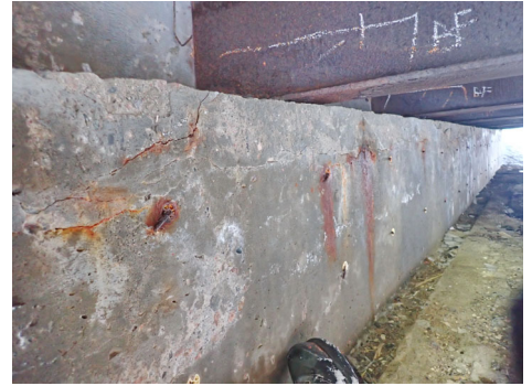
SU2 Abutment wall. Note: Typical delamination and rust staining.
