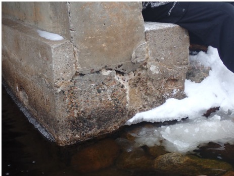
Inlet - SW corner. Note: Disintegration of footing
