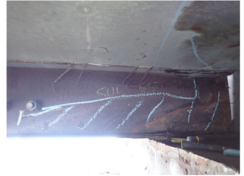
G5 @ SU1. Note: Typical corrosion.
