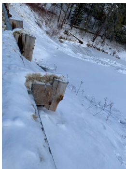
Approach Railing - SW. Note: Broken blocking at Post 4.
