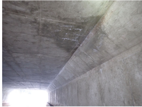
Culvert Soffit near Inlet. Note: Isolated active wet area with hairline cracks.
