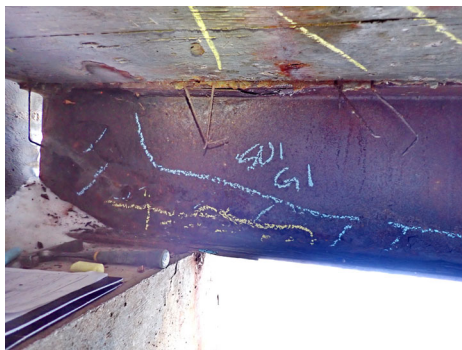
G1 @ SU1. Note: Typical corrosion.
