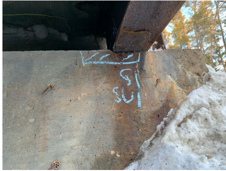
SU1 Abutment wall. Note: Spall below G1.
