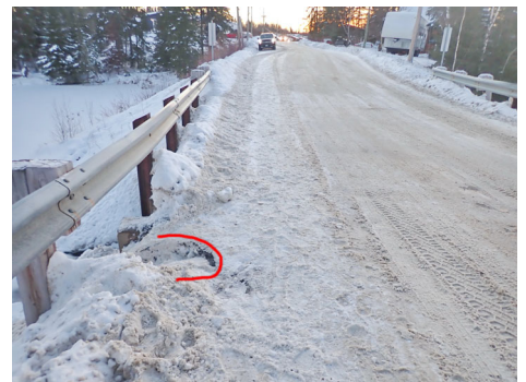
Approaches - Wearing surface - SE. Note: Missing asphalt encroaching travel lane.
