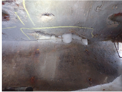
Deck Soffit - Interior - SU1 between G1/G2. Note: Spall and temporary repair.
