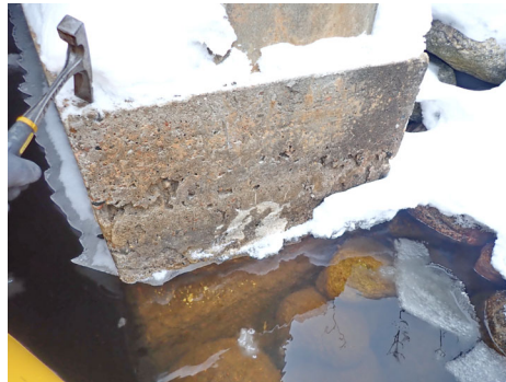
Outlet - NE corner. Note: Disintegration and erosion of concrete footing.
