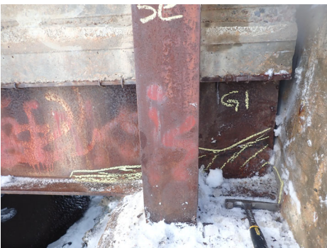
G1 @ SU1. Note: Medium corrosion on web.
