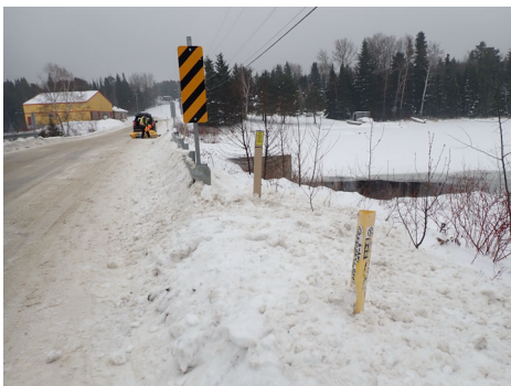
NW embankment. Note: Natural gas pipeline and cathodic protection markers.
