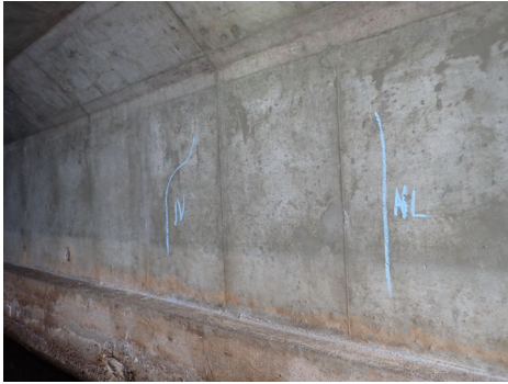
Culvert Barrel - South wall. Note typical vertical cracks.
