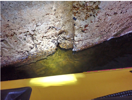
Culvert North Footing at midspan. Note: Disintegration (~400mm deep) of footing with exposed rebar.
