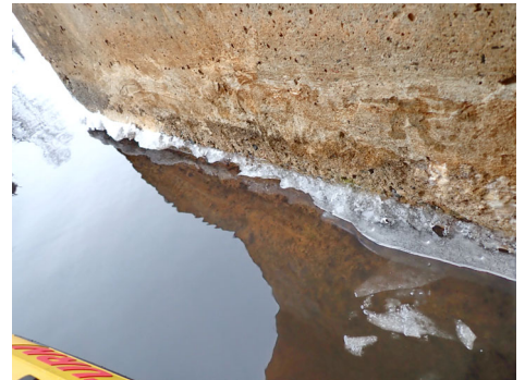
Culvert South Footing. Note: Disintegration and erosion of concrete footing with exposed rebar.
