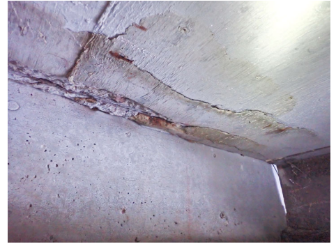
Deck Soffit - Interior - SU2 between G4/G5. Note: Typical delamination, spall, and exposed rebar.
