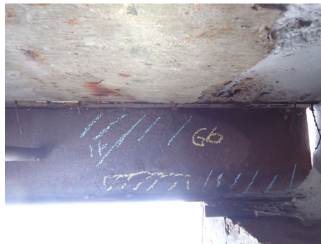
G6 @ SU1. Note: Medium to severe corrosion on web.
