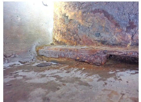
Typical interior bearing - SU1.
