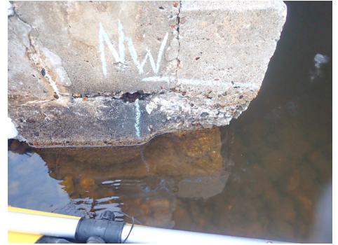
Inlet - NW corner. Note: Disintegration and erosion of concrete footing with exposed rebar.
