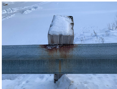
Coatings - Railing. Note: Typical rusting.
